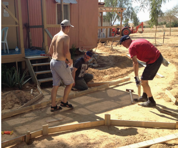
The men are laying out the concrete paths by the buildings...
